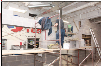
Construction on the expanded tool store & newly added tool crib, will be finished by January 10, 2011.
